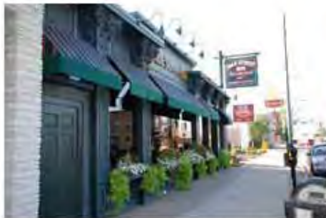
Gale Street Inn is an example of traditional main street-type retail
